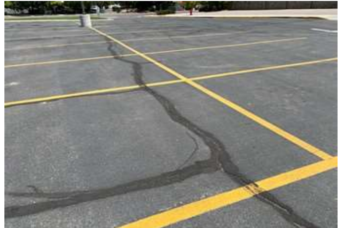
Previous crack repair
