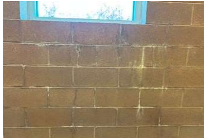
Efflorescence and cracking at gym wall
