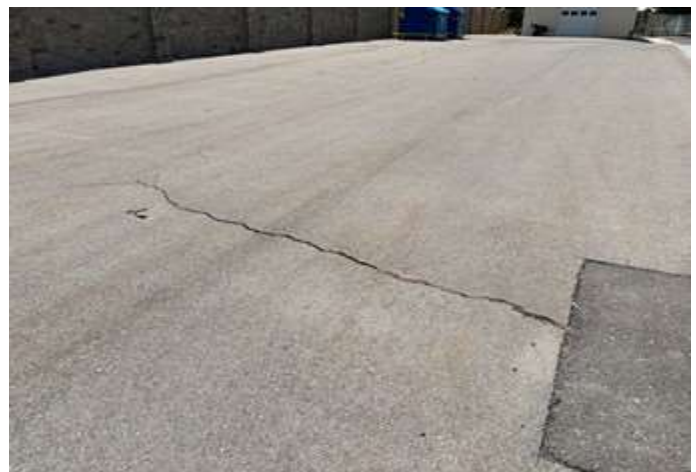
Crack in pavement near maintenance building
