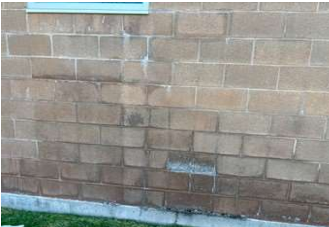
Efflorescence present
