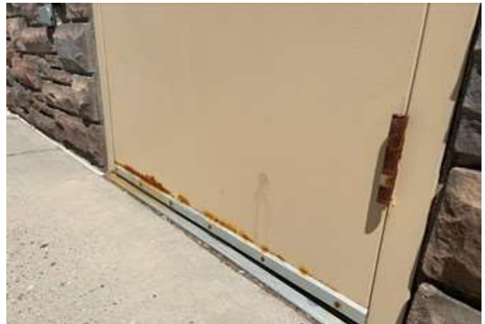
Significant rust on door and hinge
