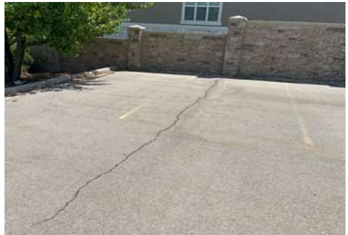
Large crack in asphalt near maintenance building
