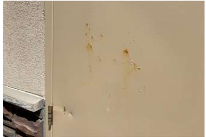
Rusted and damaged metal door
