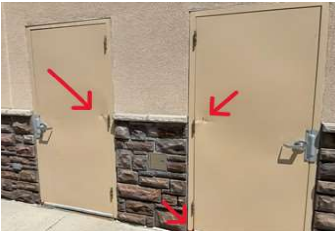
Locations of damage or rust on exterior metal doors
