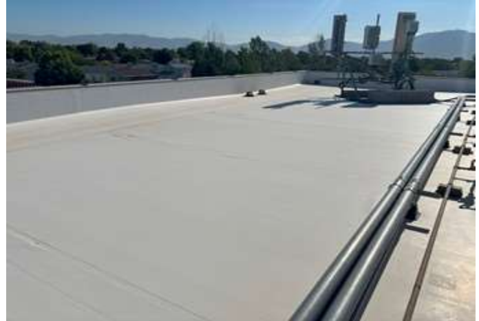
TPO roof dating to 2012
