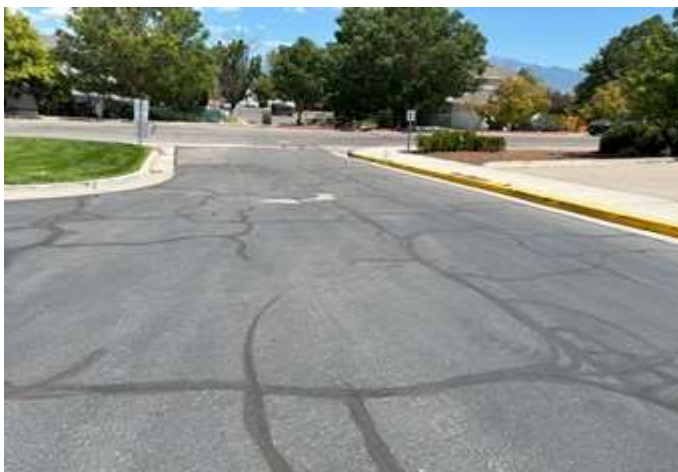
Previous crack repair
