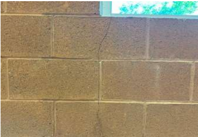
Crack in masonry
