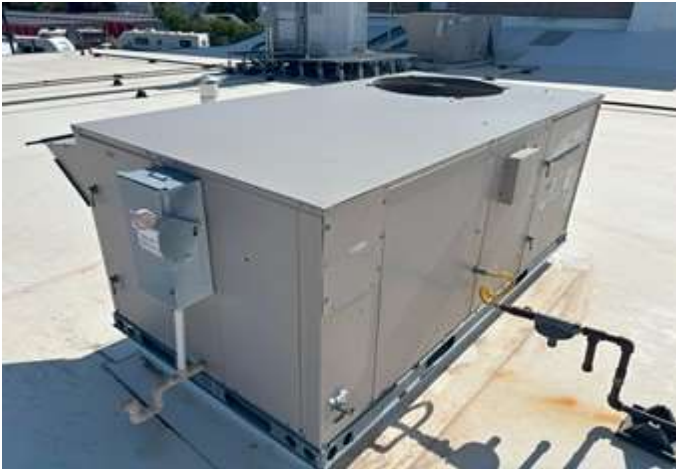
Overview of smaller rooftop unit (4 to 6 ton)
