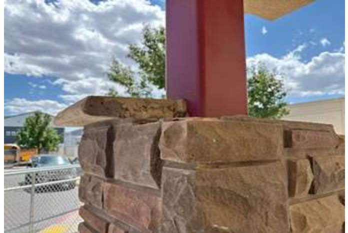
Damaged masonry at cafeteria entrance
