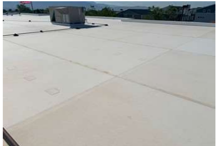
TPO roofing membrane detail
