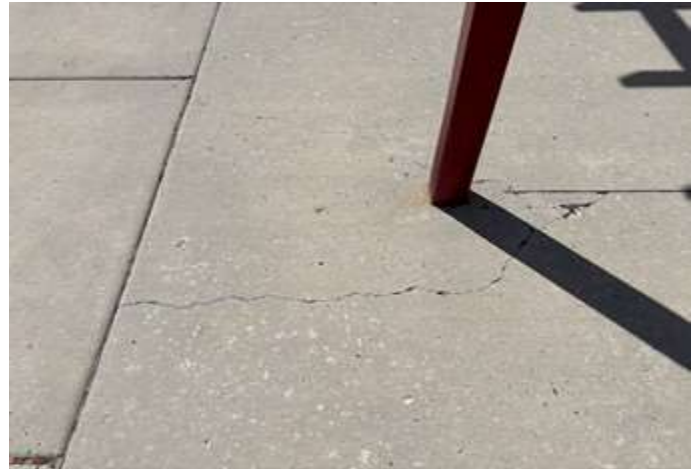
Crack in sidewalk
