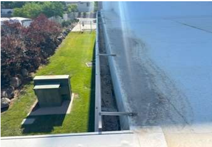
TPO roofing membrane and gutter
