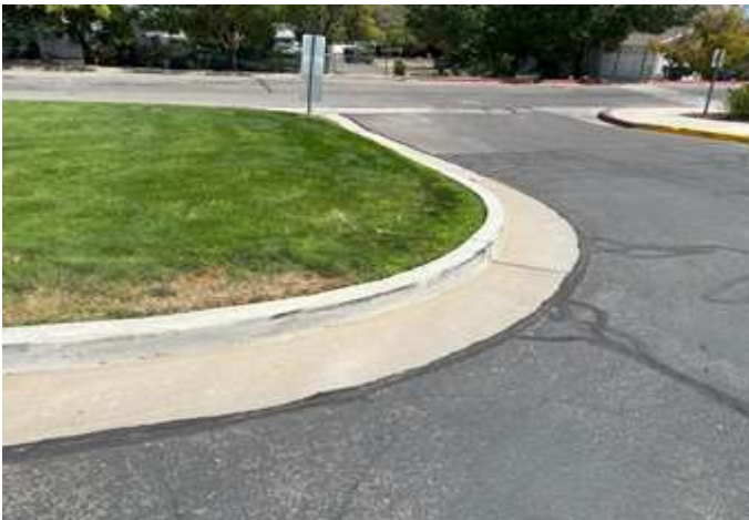
Curb and gutter in good condition
