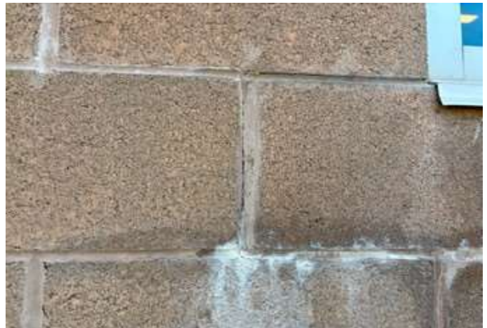
Aging mortar and efflorescence present
