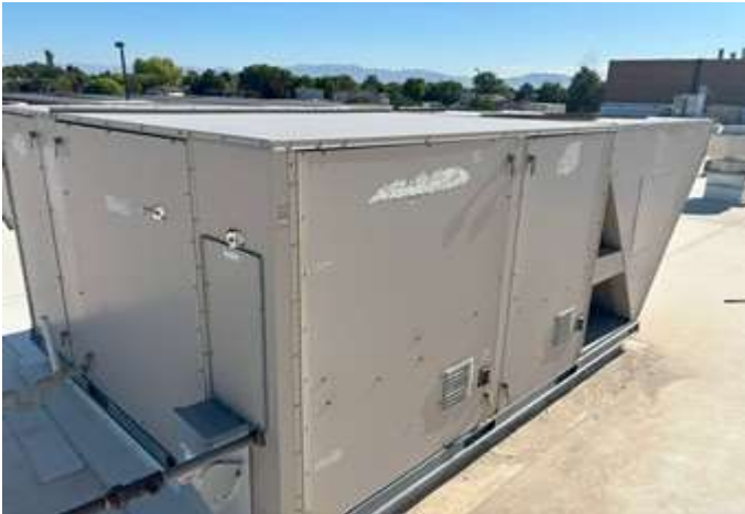
Overview of large rooftop unit (20 tons)
